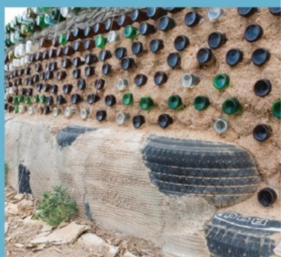
Glass bottles and old tires used in the construction of the Earthship wall ▲
